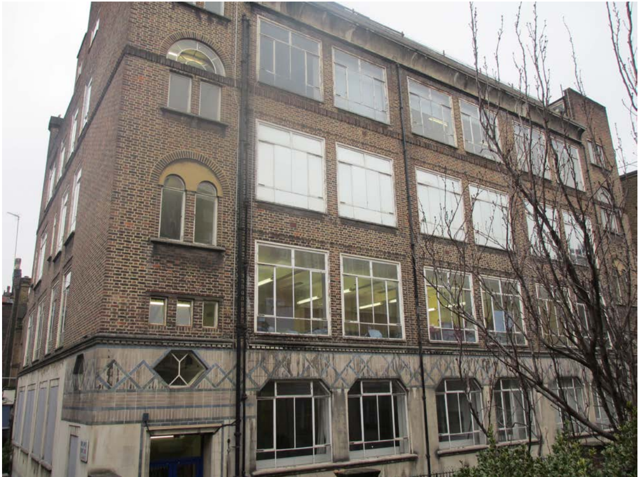
Former Westminster College building (now demolished)
